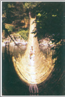
Figure 6.7 : Rope Bridge (Arunachal Pradesh)
